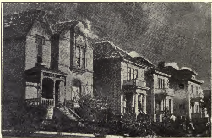
A FIRE SPREADING FROM ROOF TO ROOF
